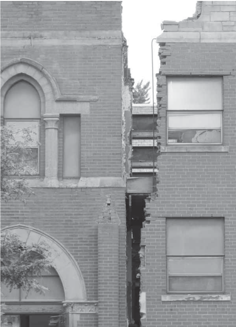
PHOTO BY BRENDA THEURER Thursday, August 13, 2026; Northwest corner of Pearl and Memphis: The demolition company's process of trying to separate St. Luke's United Church of Christ's 1903 church building on the left from the 1925 addition—with the parlor, offices and classrooms—on the right. The iconic structure faces Pearl Rd.
