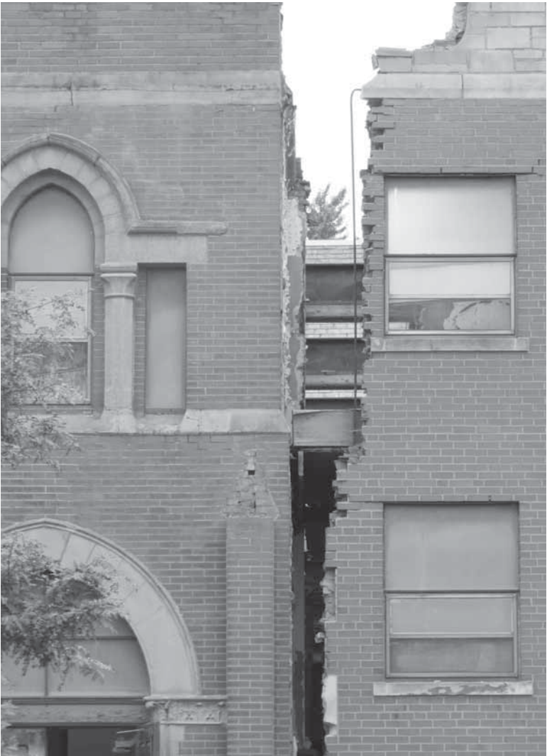
PHOTO BY BRENDA THEURER Thursday, August 13, 2026; Northwest corner of Pearl and Memphis: The demolition company's process of trying to separate St. Luke's United Church of Christ's 1903 church building on the left from the 1925 addition—with the parlor, offices and classrooms—on the right. The iconic structure faces Pearl Rd.
