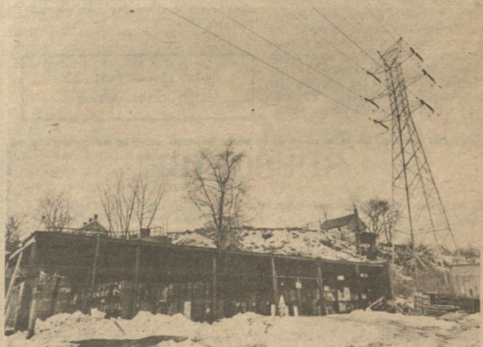
City and state officials are concerned about this chemical waste storage site located close to Tremont residential areas.
